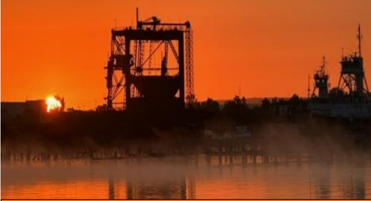
UE Local 106 Port Reading NJ. Buckeye pipeline
